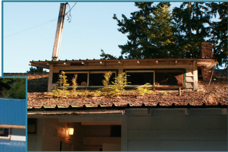
Dining hall roof before and after – notice the trees growing out of the shingles on the old roof!
